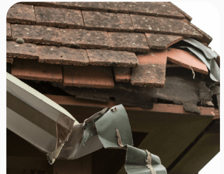
Roof, windows and gutters
